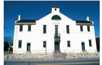
Gates County Courthouse, 1836 (NCAOC file photo)
